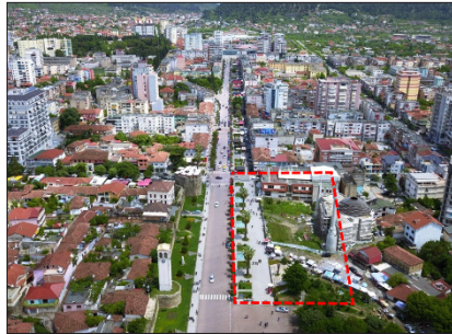
Figure 24: The bazaar site, which is now a plaza
