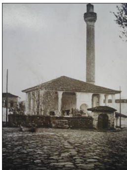
Figure 18: The original Pasha Mosque (Photo: https://www.facebook.com/photo/?fbid=2382816198672070&set=a.1438818959738470 )
